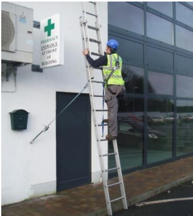
Temporary Ladder restrained in position
