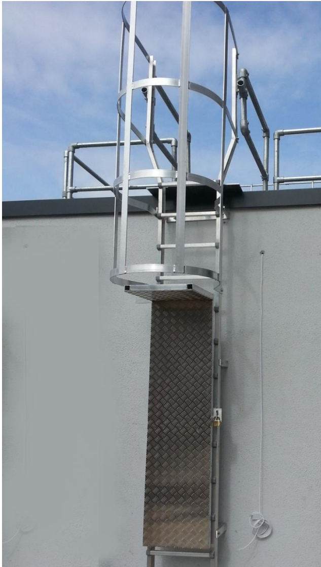
Fixed Vertical Ladder
